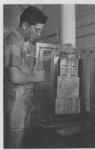
ETCHING the excess copper from the laminate is done by ferric chloride acid spray inside the tank by Dick Chavez. Both sides of the circuit card will be etched simultaneously.
